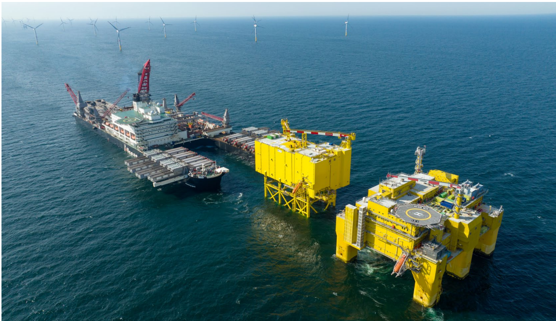
Installation of the DolWin kappa topsides by Pioneering Spirit
