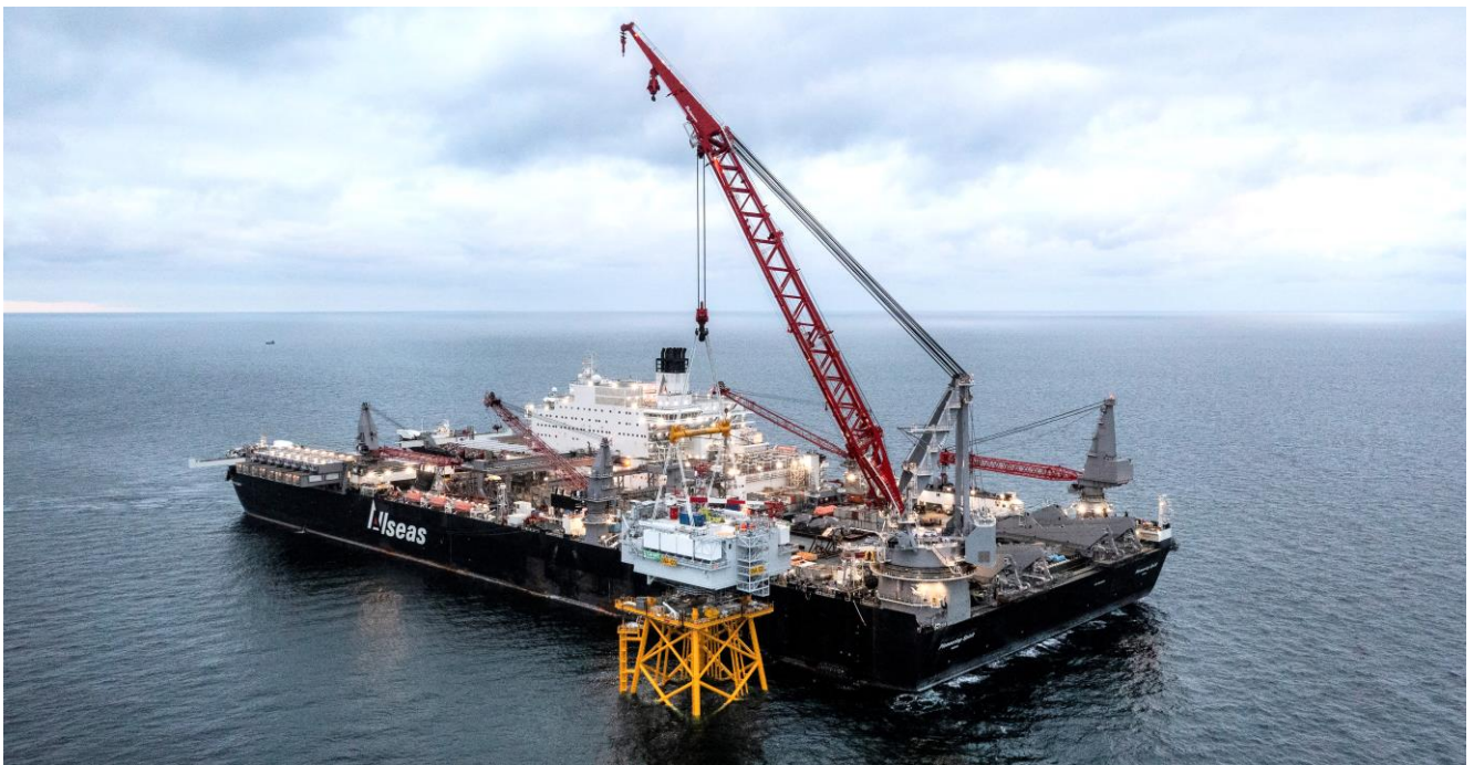
Pioneering Spirit lifts the substation into place
