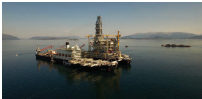
Topsides seafastened ready for the voyage.
