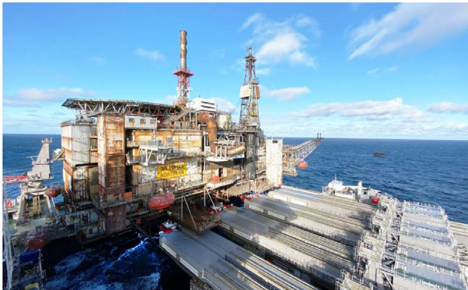
Pioneering Spirit completes the single-lift removal of 14,200 tonne Ninian Northern topsides
