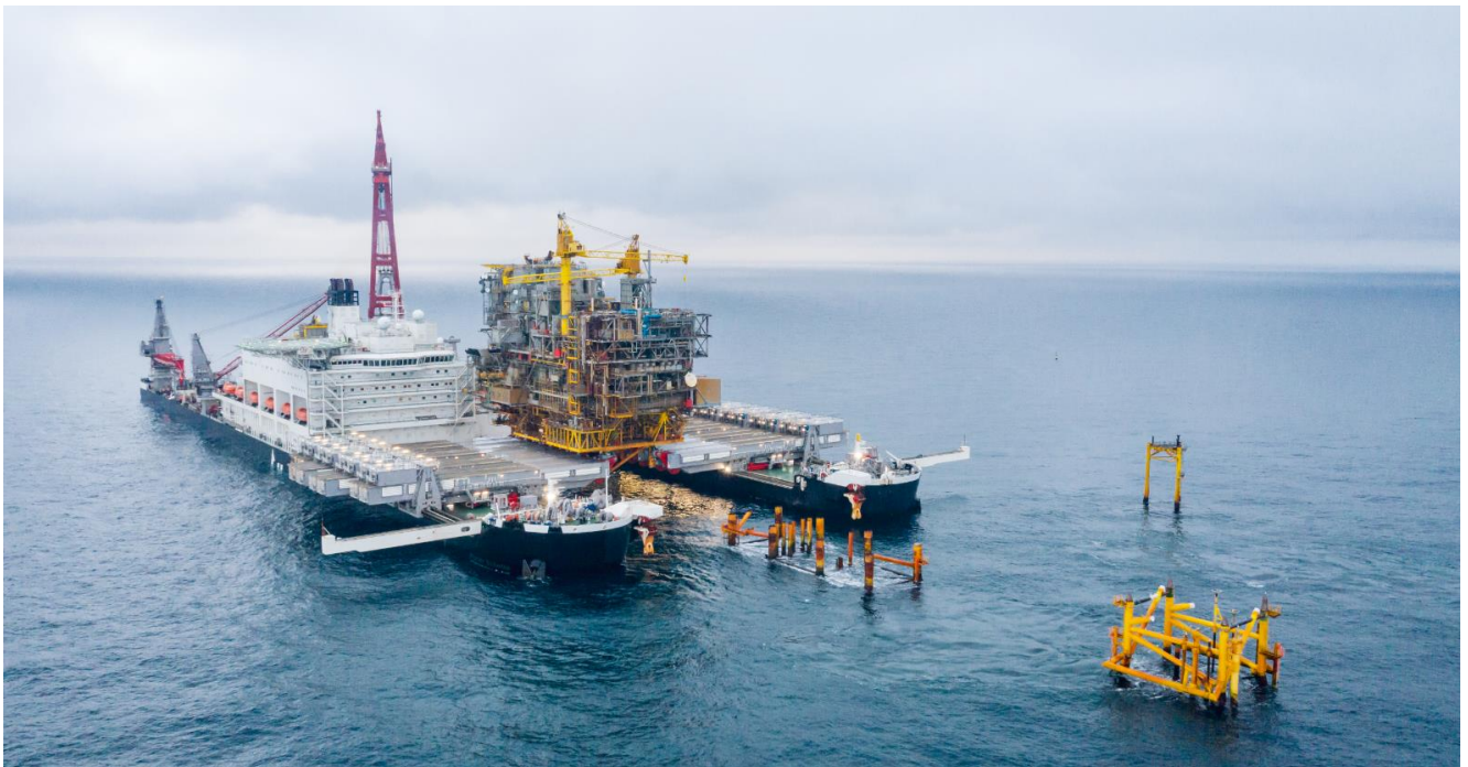
Single-lift removal of the 14,000 t TEA topsides by Pioneering Spirit on 2 August 2020
