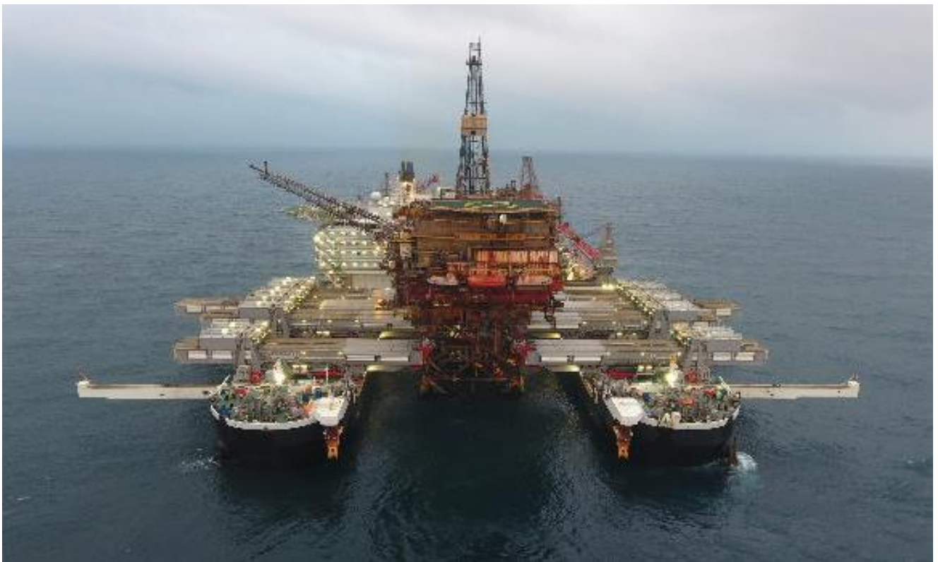
Ready for lift off – fast-lift of the Brent Alpha topsides
