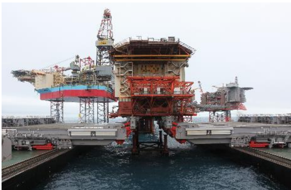
The "fast lift" of the QP topsides took only 9 seconds
