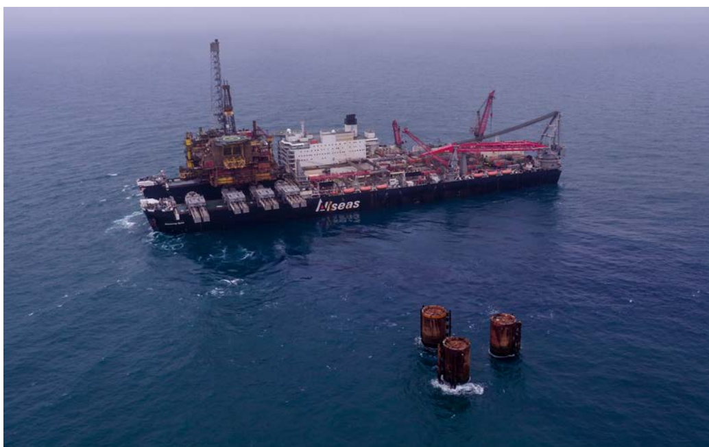
Pioneering Spirit removes 25,000 t Bravo platform
