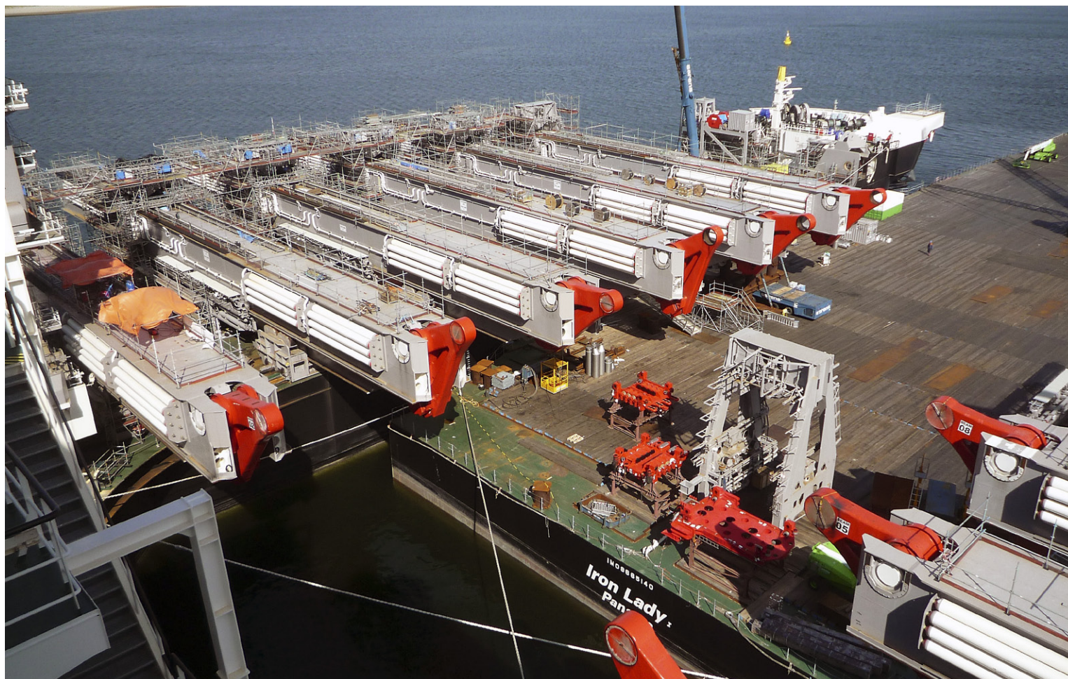
FILLING THE SLOT: Transport barge Iron Lady has provided a working surface for beam installation work
