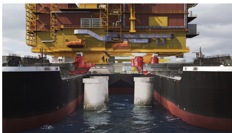
YOKE OPTION: The first two contracts will employ yoke connectors, as illustrated here pushing up beneath a topside just after completion of the fast lift at a concrete gravity base.
