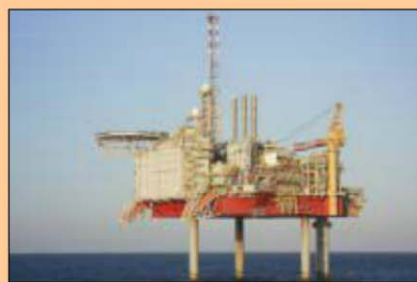
Condemned: the Yme platform
