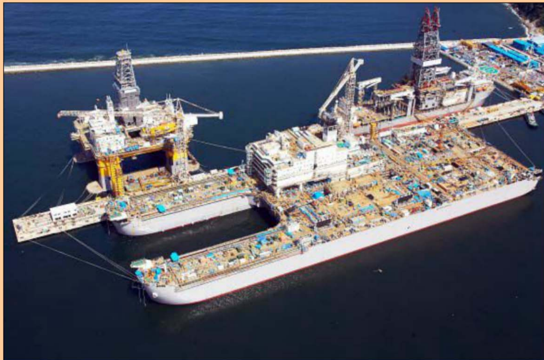
Giant in demand: Allseas' Pieter Schelte under construction at Daewoo
